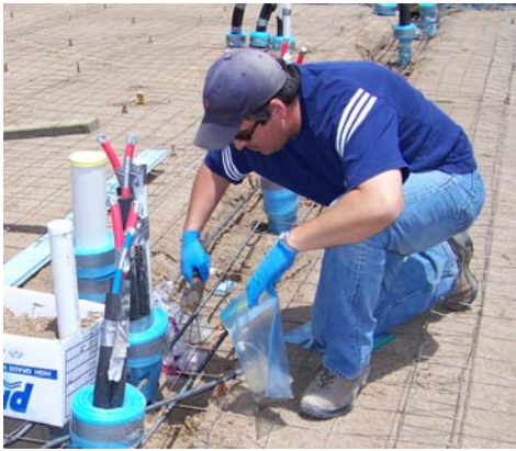
Termiticide Application Inspection
